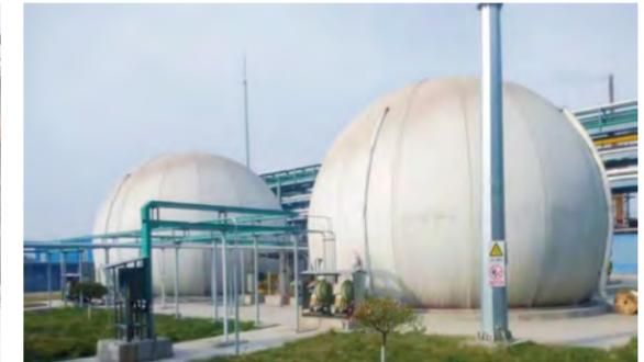
We utilize the biogas generated during the wastewater treatment process as fuel for the hot air furnace, reducing the use of natural gas, effectively promoting resource recycling and mitigating the impact on the environment.
